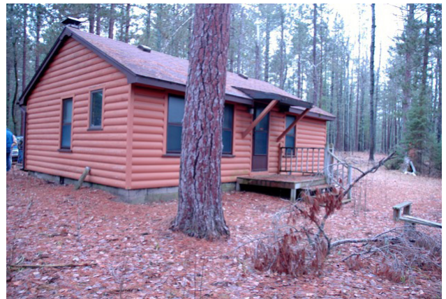
Half-log structure off Sawdust Pile, a candidate for proposed rental program.
