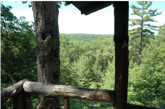
View from Honeymoon Cabin porch that's now considered unsafe.
