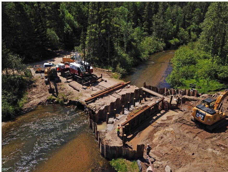
Three cylinders known locally as the tubes were replaced this spring with abutments for a new timber bridge over the Pigeon River (flowing right to left in this view) at the east end of Ford Road. Photo by Dutch Neubecker
