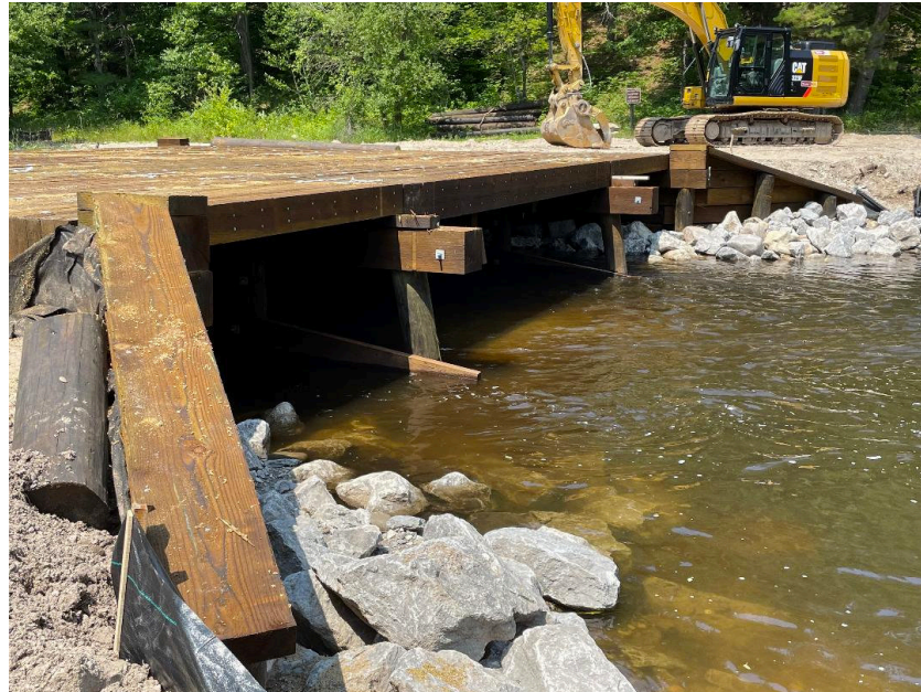
The Otsego County Road Commission assembled the deck after contract work, supervised by Josh Leisen, Huron Pines senior project manager, removed the cylinders. Photo by Sandra Franz
