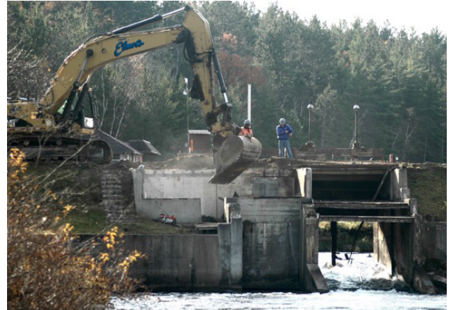
The entire dam structure began coming down on October 26.
