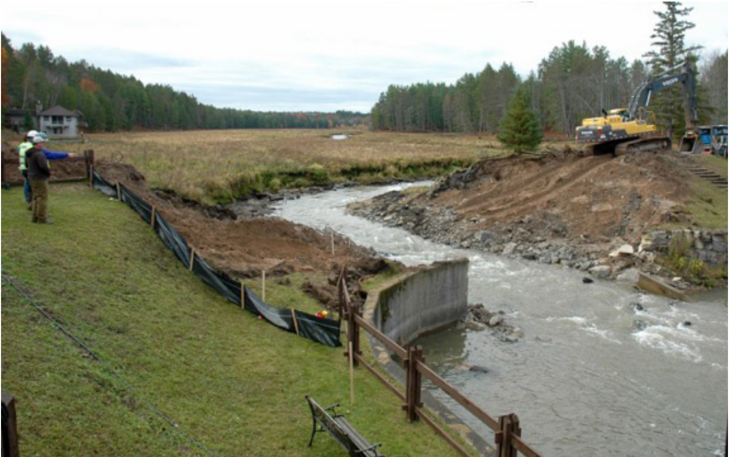
The Pigeon River flows unimpeded through the deconstructed Song of the Morning dam (exits on bottom right). The former pond, now vegetated, is in the center of the photo. @ Dale Franz
