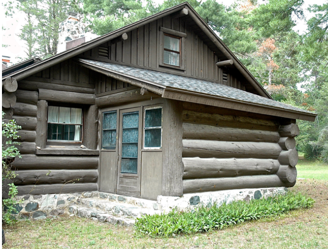
Back door before walkway was discovered this summer at Discovery Center.
