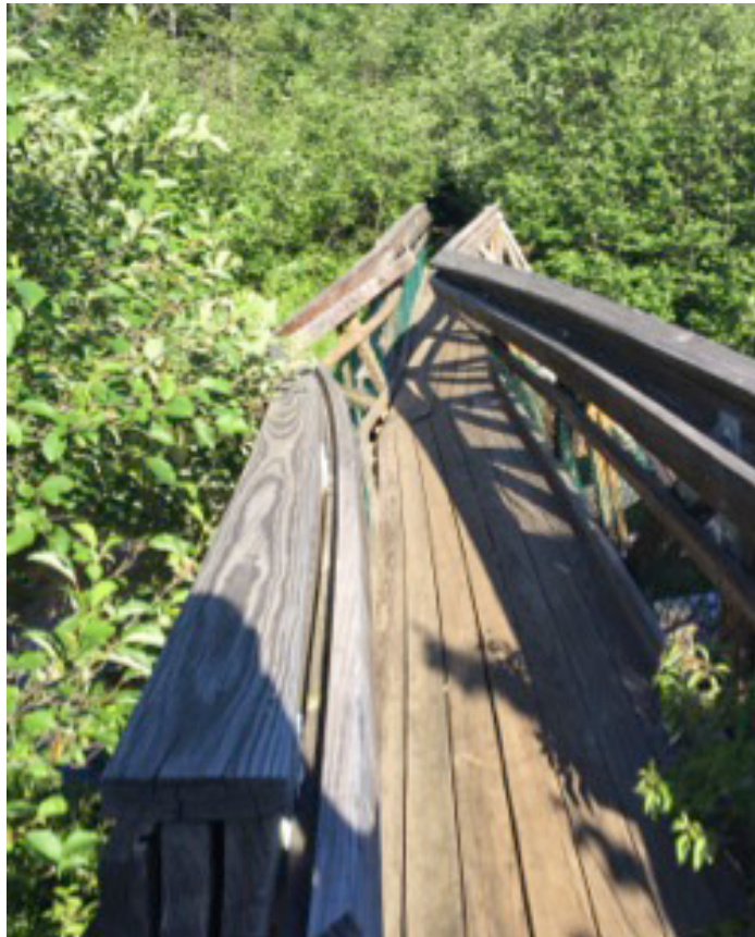
Bridge over Black River. (DNR photo)
