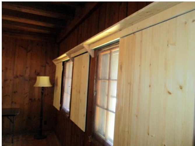
Volunteers built three wooden sliders to cover windows when showing images on a screen in one room of the Discovery Center. @ Rudi Edel
