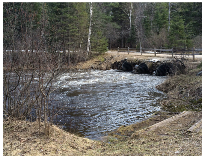
Plunge pool at outflow of culverts will get shallower as the artificial velocity of the water slows to natural flow. Photo by Lisha Ramsdell
