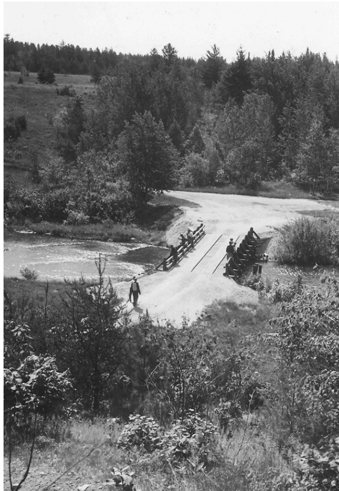
This 1940 photo shows the wooden bridge that preceded the embankment and culverts that will now be replaced. The Pigeon flows right to left in the image.
