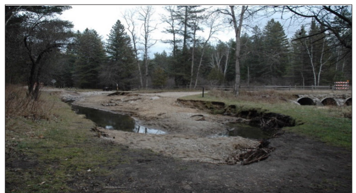
Campsite 19 at Ford Lake Road was washed away by Pigeon River during a late October 2020 rainstorm. Water approaching tubes overflowed bank shown here on right.
